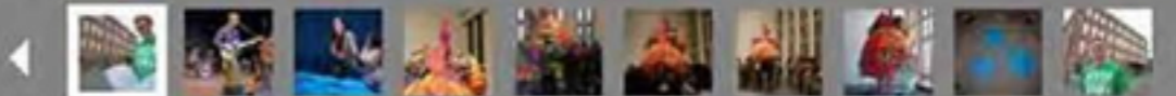
Jeff Mirel of The Albany Barn stands in front of the abandoned St. Joseph's Academy which The Albany Barn will be transforming into art space and studio apartments on North Swan St. in Albany, N.Y. Wednesday, Sept. 21, 2011. (Lori Van Buren / Times Union) (Albany Times Union)
